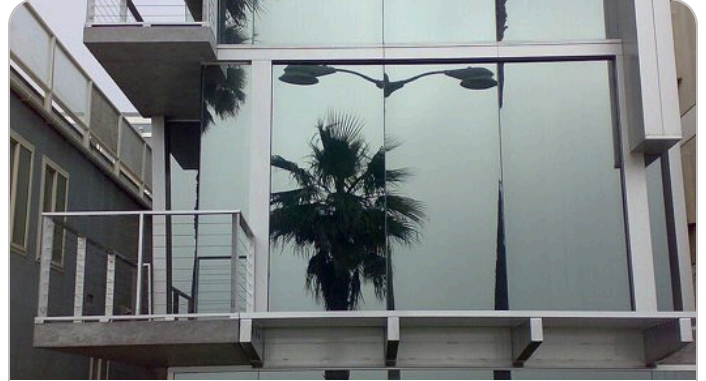
Building envelope: glazing and shading Photo: Jon Rawlinson • CC BY 2.0 • source
