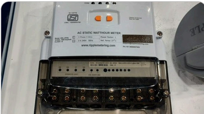
Three-phase energy meter — records kWh, and kVA maximum demand over 30-minute windows
