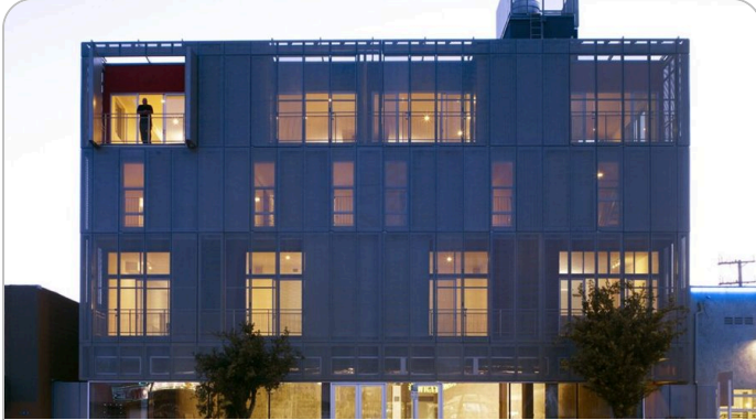
Office façade — window-wall ratio, SHGC and VLT of the glazing decide the cooling load and daylight Photo: Calderoliver • CC BY-SA 3.0 • source
