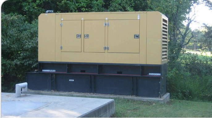
Packaged diesel generator set in an acoustic enclosure
